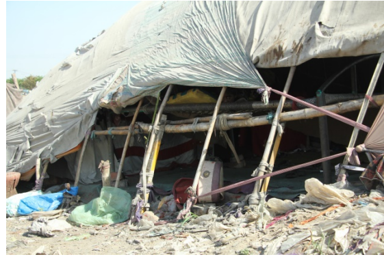
Fig. VIII. Representing the bamboo structure for hut and cloth used as covering in summers
